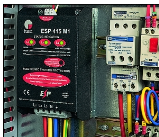
ESP 415 M1 installed within a control panel on the mains input to protect the panel's control systems. Note the remote indication connection (top of protector).
